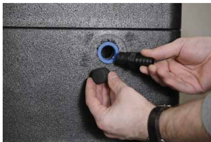
Connecting the condensate drain
