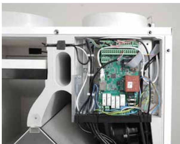
Remove control board
