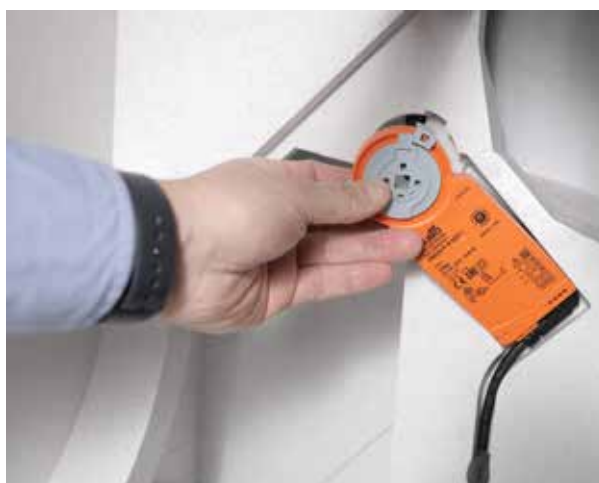
Remove bypass actuator
