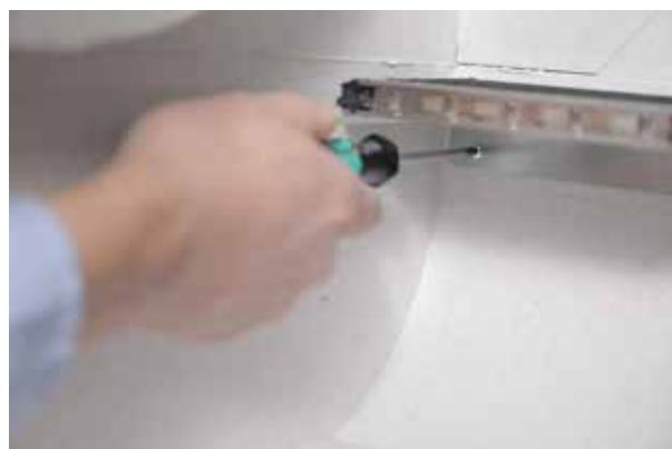
Remove built-in electric preheating surface (optional)
