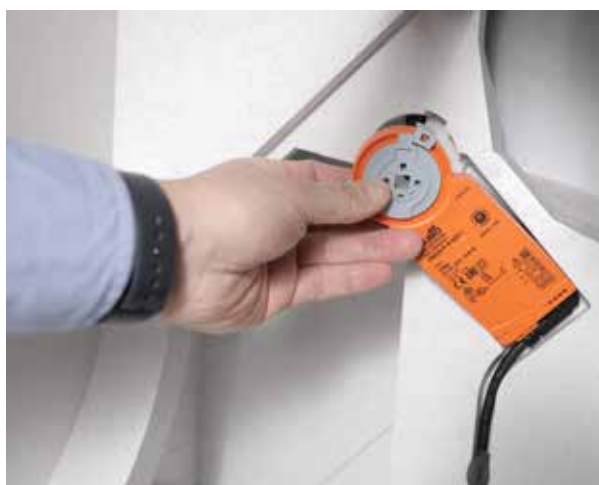
Remove bypass actuator
