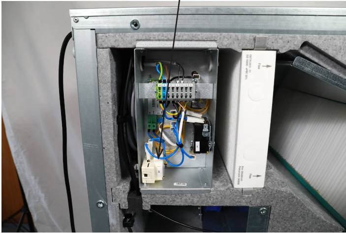
Built-in electric heating surface in ECO 400 XL
