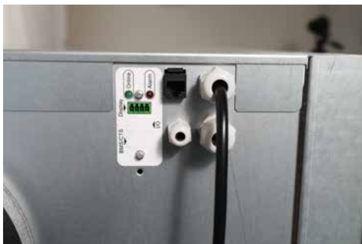
Connections for the Internet, display, CTS and accessories on ECO 400 XL
