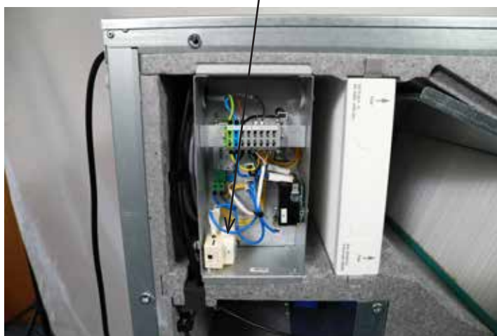
Built-in electric heating surface in ECO 400 XL
