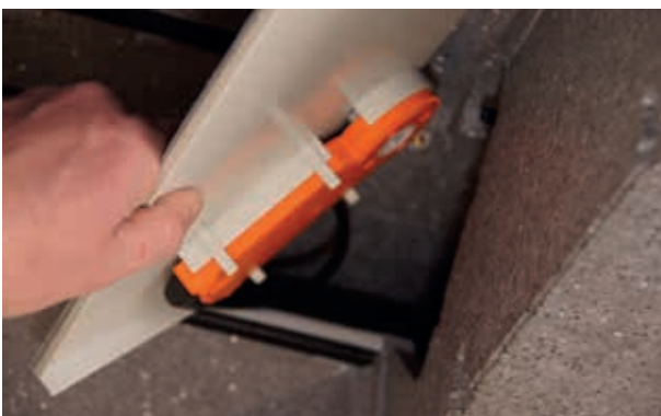
Remove bypass actuator
