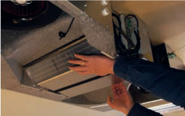
Remove heat exchanger
